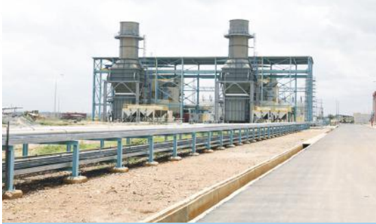
KTPS 220MW Thermal Plant
