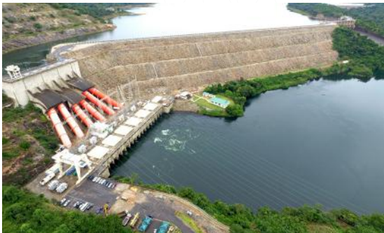
Akosombo Dam 1020MW Hydro Plant
