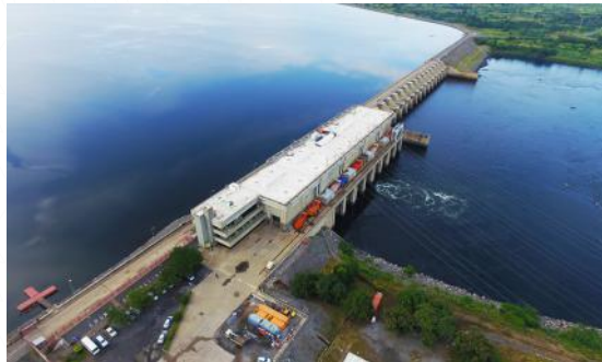
Kpong Dam 160MW Hydro Plant
