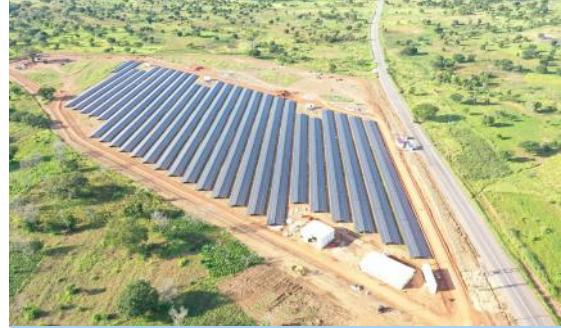
6.5MWp Lawra Solar Power Plant
