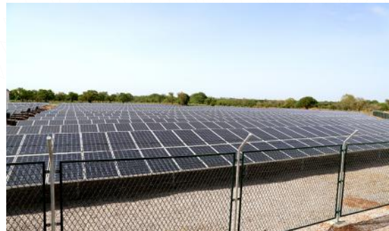
2.5 MWp Navrongo Solar Power Plant
