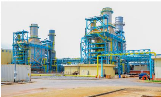
330MW Takoradi Thermal Power Station (TAPCo -T1), Aboadze
